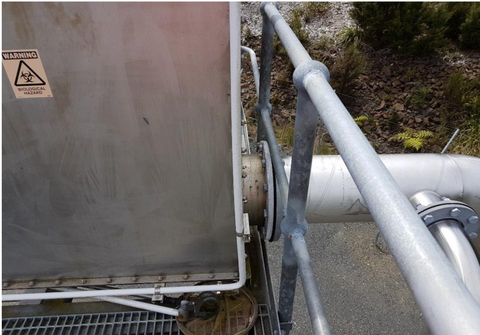
**Figure 2: Mangawhai WWTP Inlet Screen.**
