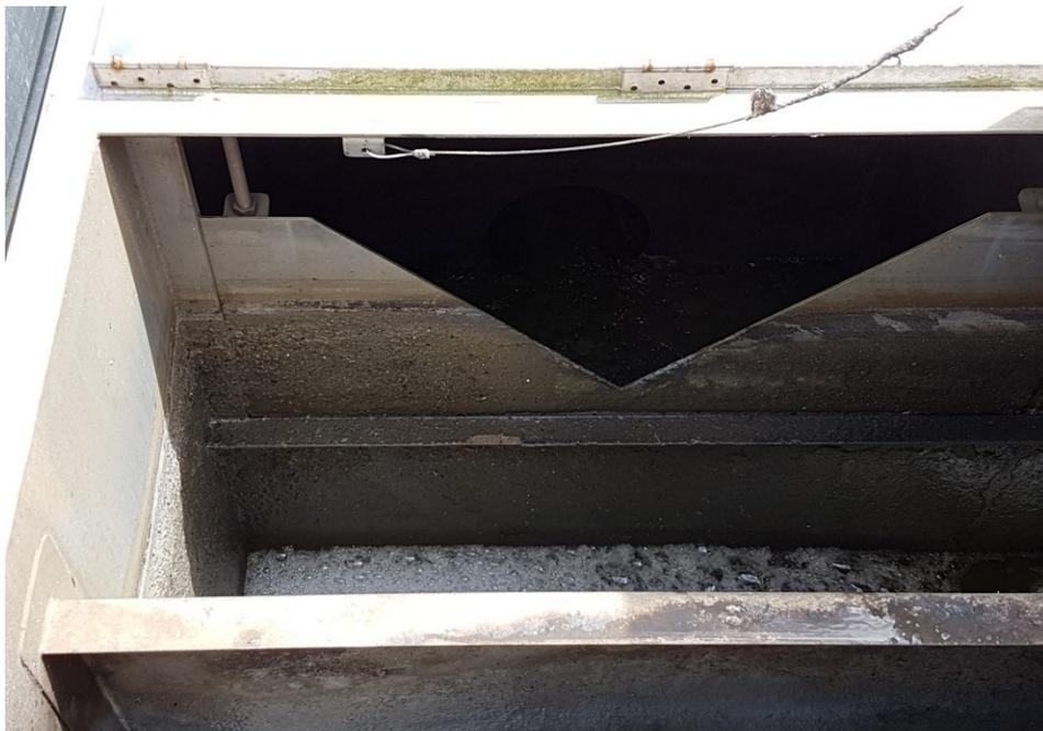
**Figure 3: Splitter box internal view**
