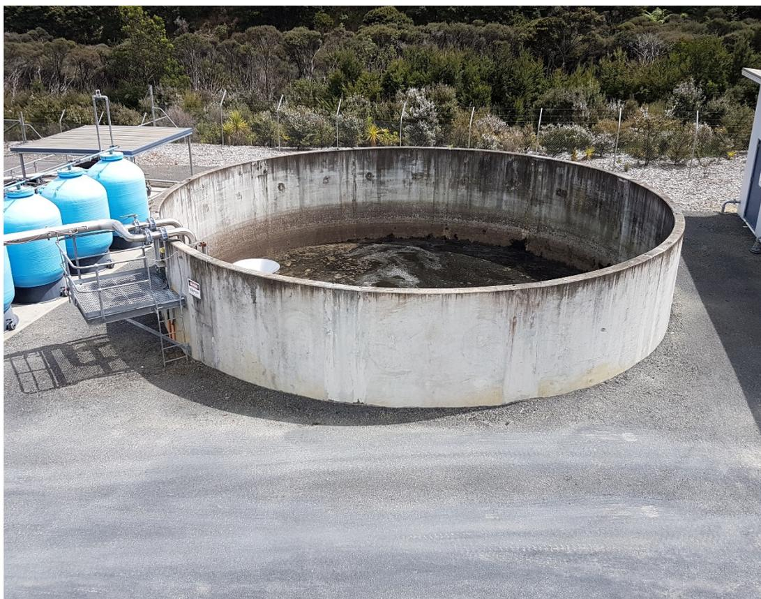
**Figure 6: Intermediate Storage Tank located downstream the CASS System**
