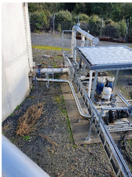
Figure 5 Current treated water pumps and wash water pumps next to the treated water tank.
