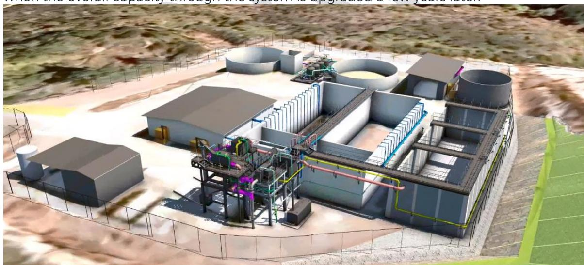
*Figure 4 : 3D Model of Mangawhai WWTP with Balance Tank*
