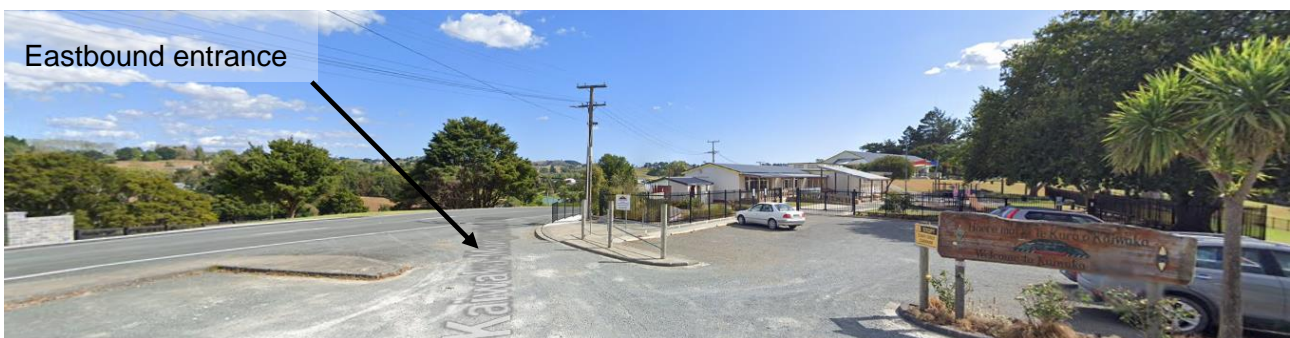
Figure 14: Kaiwaka School – eastern entrance to main carpark and staff carpark
