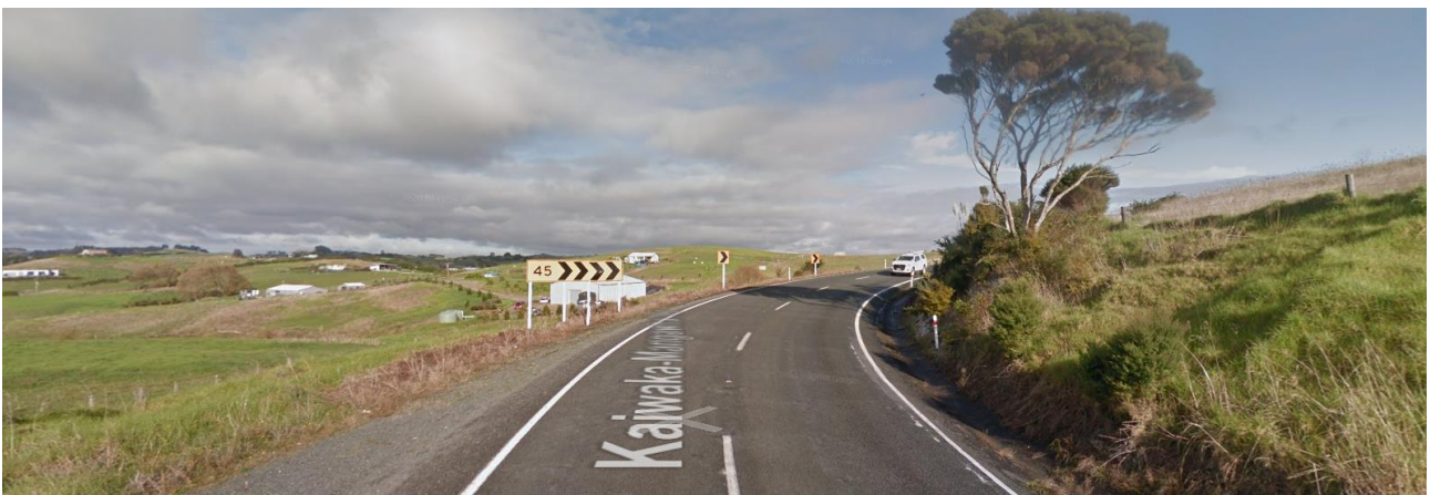
Figure 35: Kaiwaka-Mangawhai Road – low advisory speeds for curves with limited visibility.
