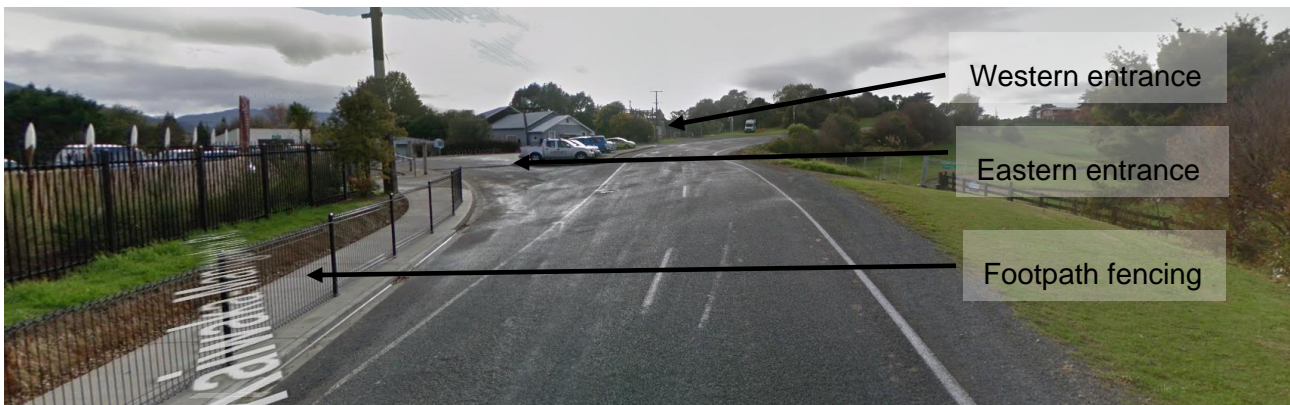
Figure 12: Kaiwaka School entry - eastbound
