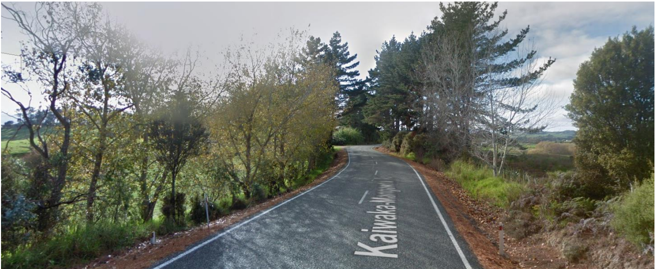
Figure 34: Kaiwaka-Mangawhai Road – narrow shoulder widths typical of this road
