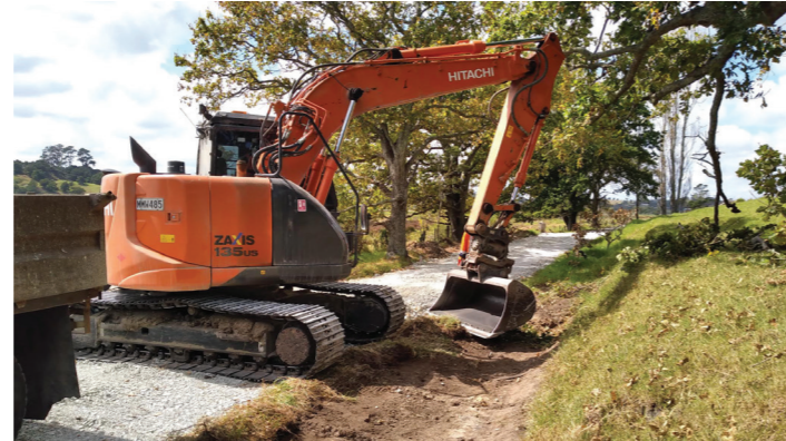
Work started on Kaihu Valley Trail
