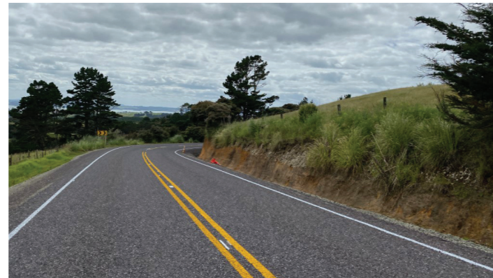
Poutō Road phase 1 sealing completed
