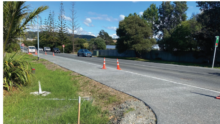
Mangawhai shared path work is progressing
