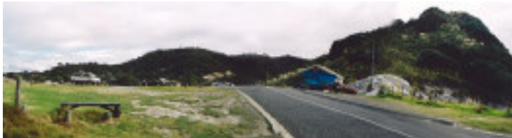
location of existing toilet block inappropriate
