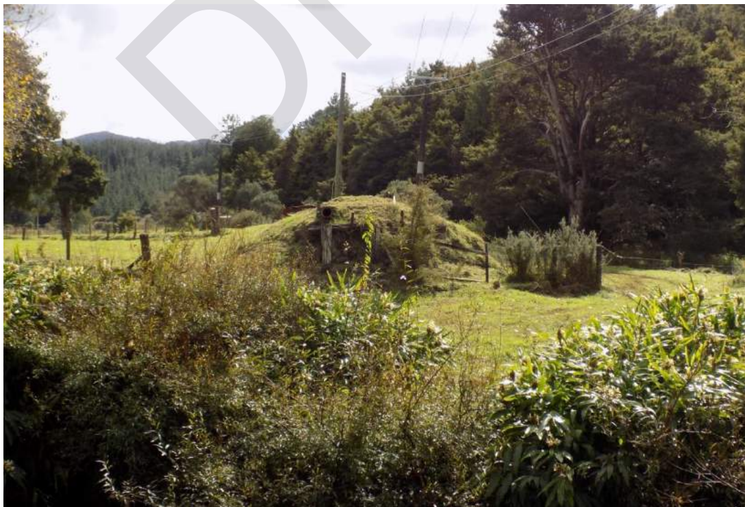
Figure 18: An image of the northern bridgehead of the Ahikiwi Bridge taken from the south side of the Kaihu River.
