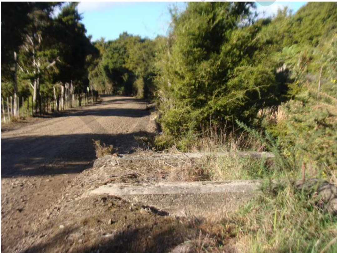
Figure 28: Looking east showing the base of the water supply tower at Tarawhati Station on the Aranga Station Road
