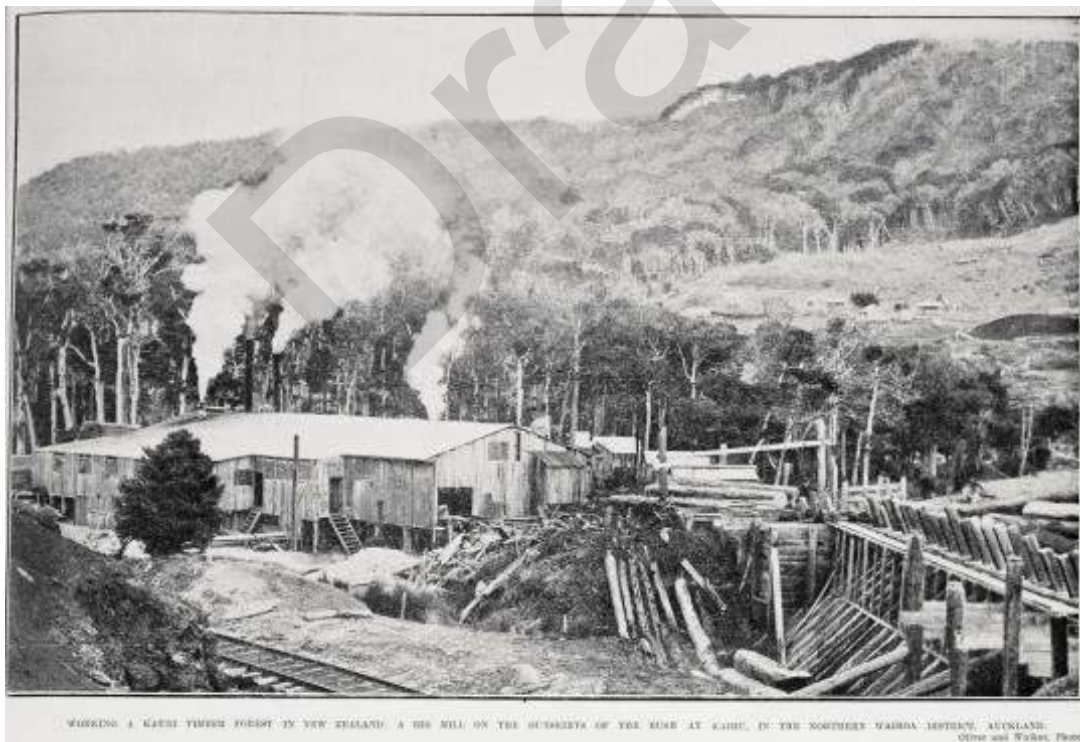
Figure 6: Trounson's sawmill at the Kaihu Booms in 1912. Note the KVR railway line. On the right of the image is a dam with logs floating in the water behind. This is where the boom, a floating barrier, that kept the logs contained ( Auckland Weekly News , 1 September 1912 p.11, Auckland Libraries Heritage Collections AWNS-19100901-11-1).
