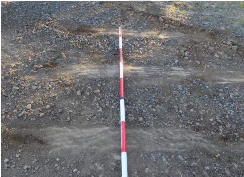
Figure 33: A sleeper feature at the very western end of Aranga Station. The sleepers are set into Aranga Station Road and have somewhat survived graders and other road workings over the years.
