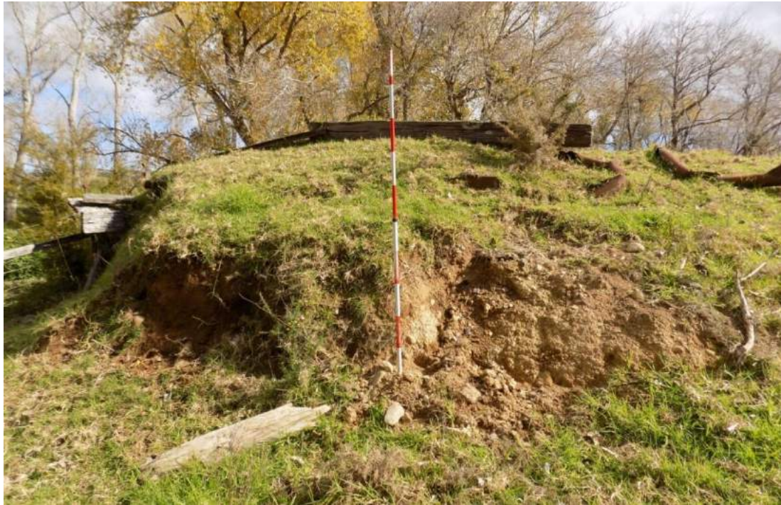
Figure 19: The southern bridgehead of the Ahikiwi Bridge. Squared timber from the bridge remains on site. Animals have been burrowing into the clay base. The bridge was swept away by cyclone Bola in 1987.
