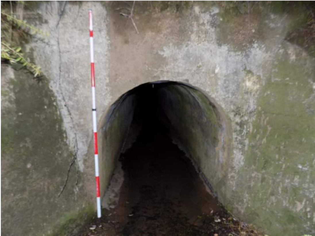
Figure 31: Concrete culvert to the south of Whatoro Station.
