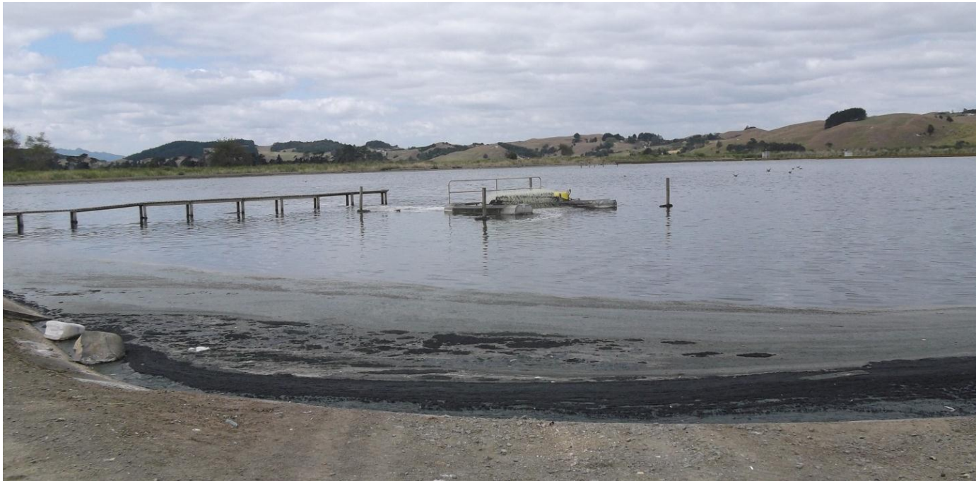
Figure 2-7 : Dargaville Treatment Plant - Oxidation Pond
