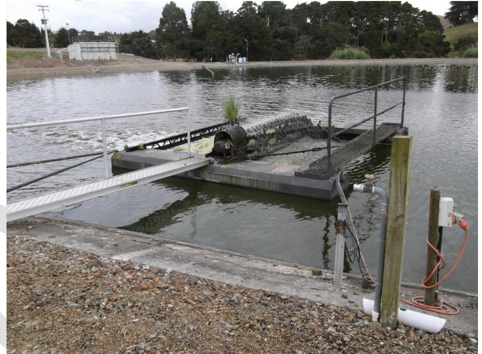
Figure 2-16 : Maungaturoto Treatment Plant – Aerator
