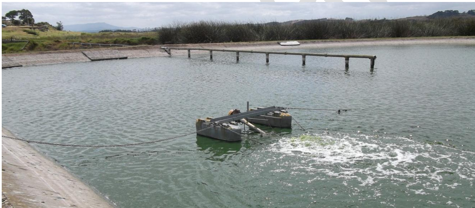
Figure 2-18: Te Kopuru Treatment Plant - Oxidation Pond
