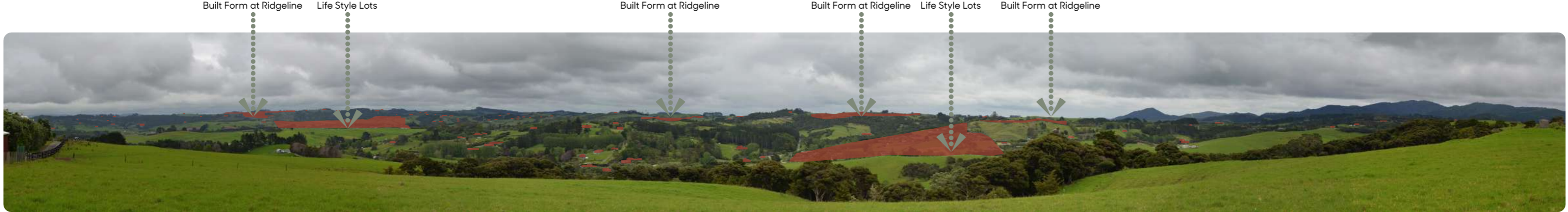
PN-02A: PANORAMA VIEW - NORTH RIDGE LINE (HIGHPOINT) OF SITE: SOUTH-WEST VIEW SHOWING BUILT FORM SITTING ACROSS LANDFORM OPPOSITE SITE
