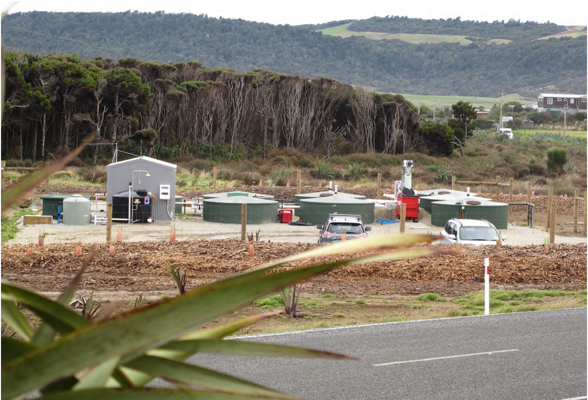
Curio Bay MBR wastewater treatment plant
