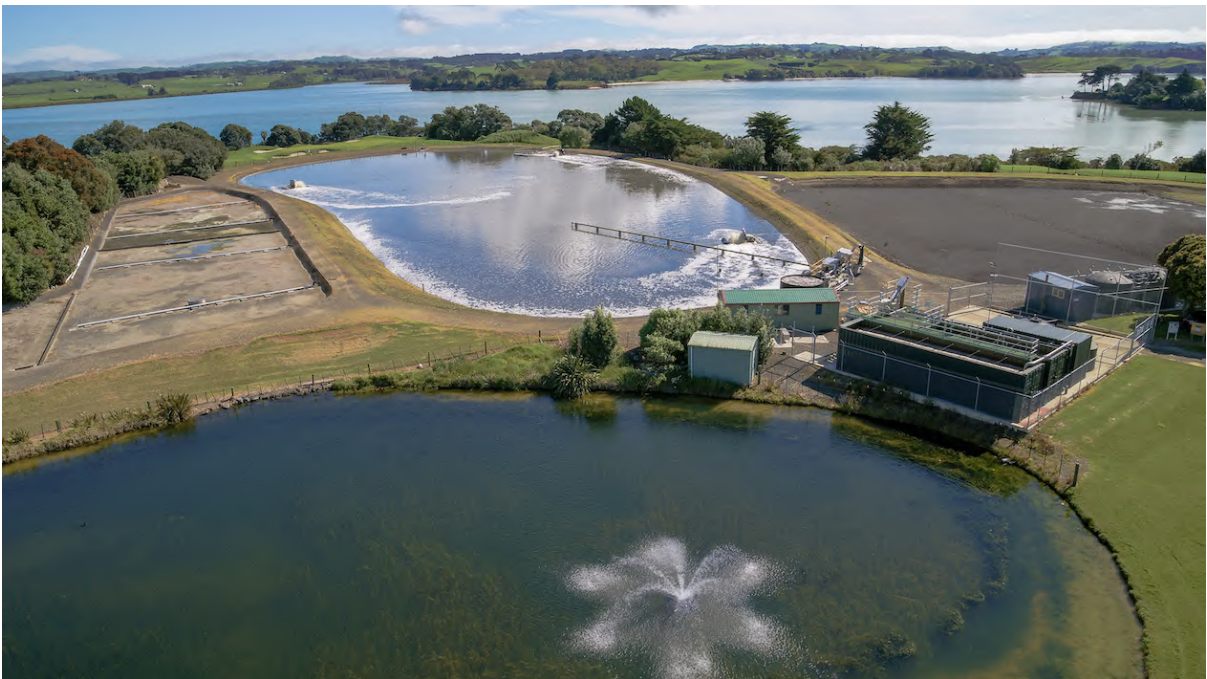
Clarks Beach MBR wastewater treatment plant upgrade
