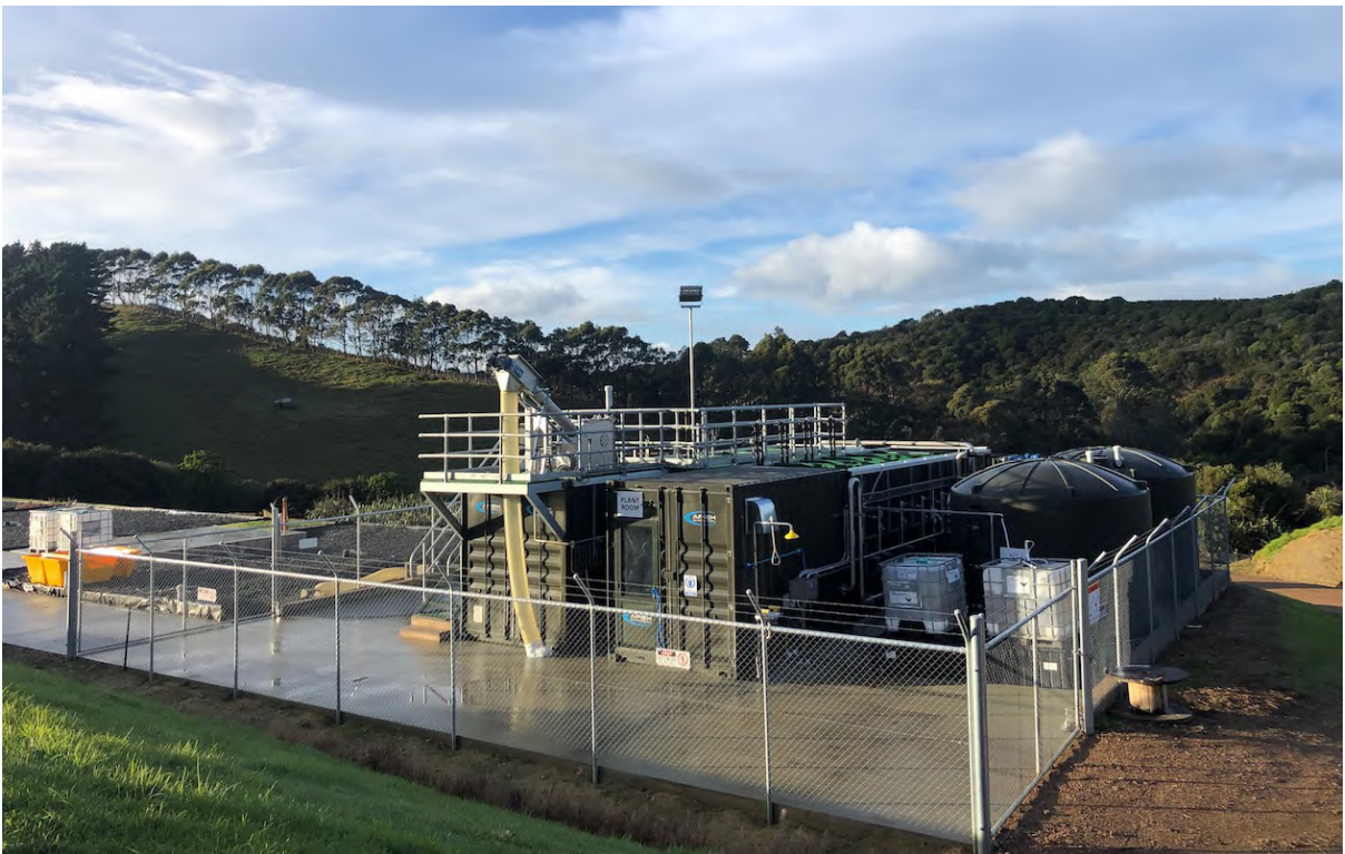
Owhanake MBR wastewater treatment plant upgrade
