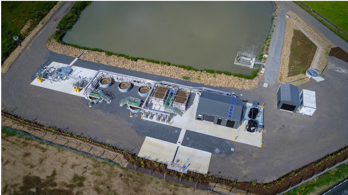
Watercare Meremere MBR wastewater treatment plant upgrade
