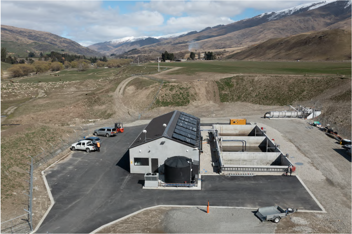
Cardrona Valley SBR wastewater treatment plant
