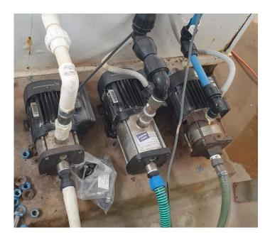
Figure 16: Chemical Carrier Pumps
