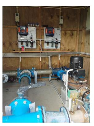
Figure 20: Final FAC and pH Analysers
