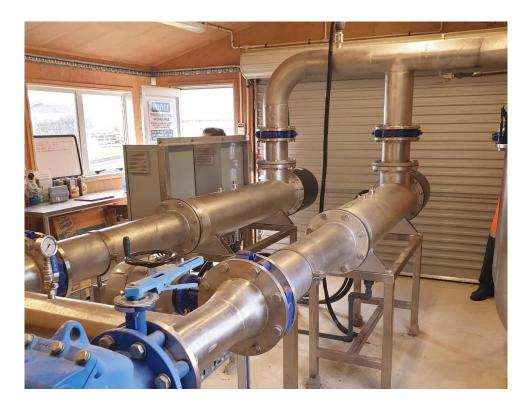
Figure 8: Duty/Standby UV Reactors
