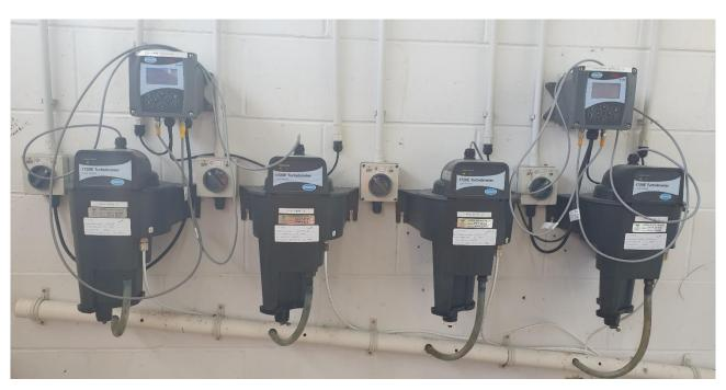
Figure 18: Turbidity Analysers and Transmitters for Filters
