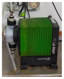
Figure 13: Alum Dosing Pump
