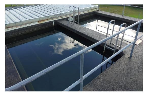
Figure 7: Two of the four Rapid Sand Filters
