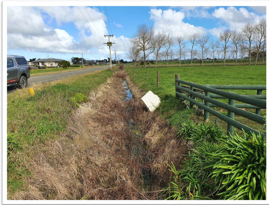
Figure 17: Picture depicting roadside table drain downstream of site
