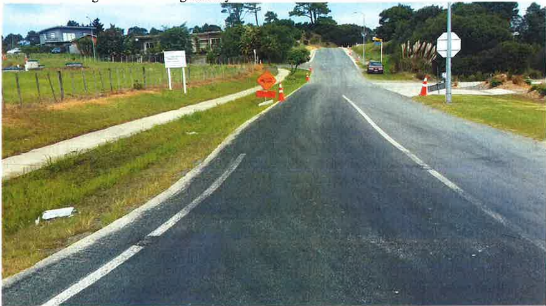
Photo 4. Looking southeast along Estuary Drive from Molesworth Drive. The site is at left.
