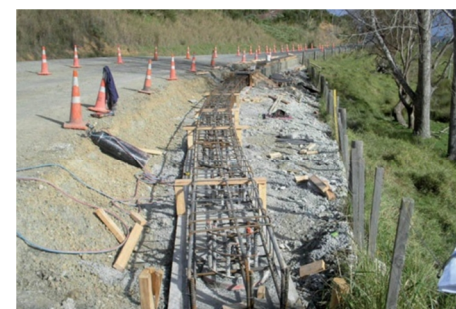
Slip Repair Works
