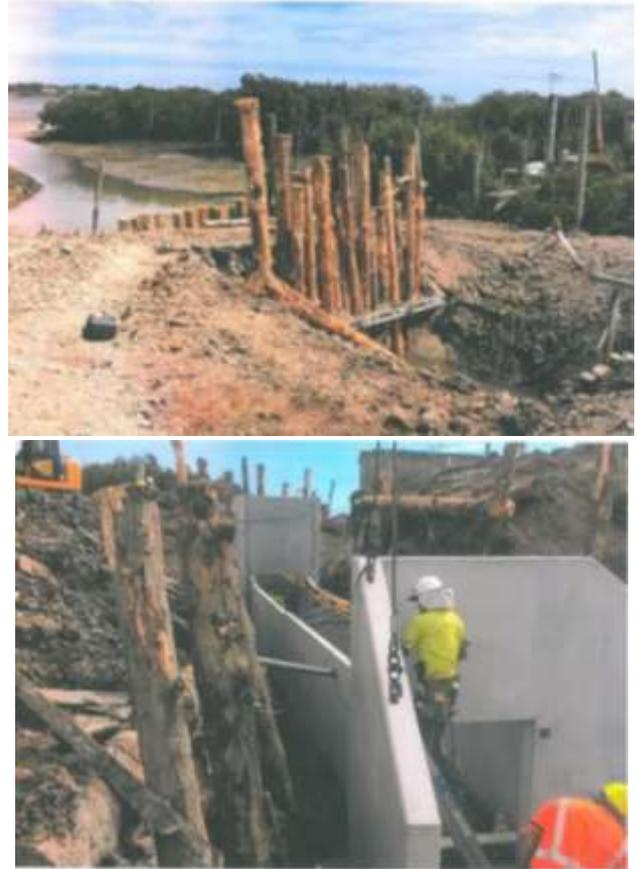
*Works carried out to undertake replacement of Floodgate N°38 on Te Kowhai Floodgate Road*
