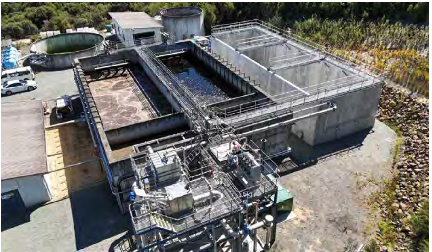
Photo: Mangawhai Wastewater treatment plant
