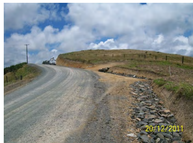
Lawrence Road Improvements after
