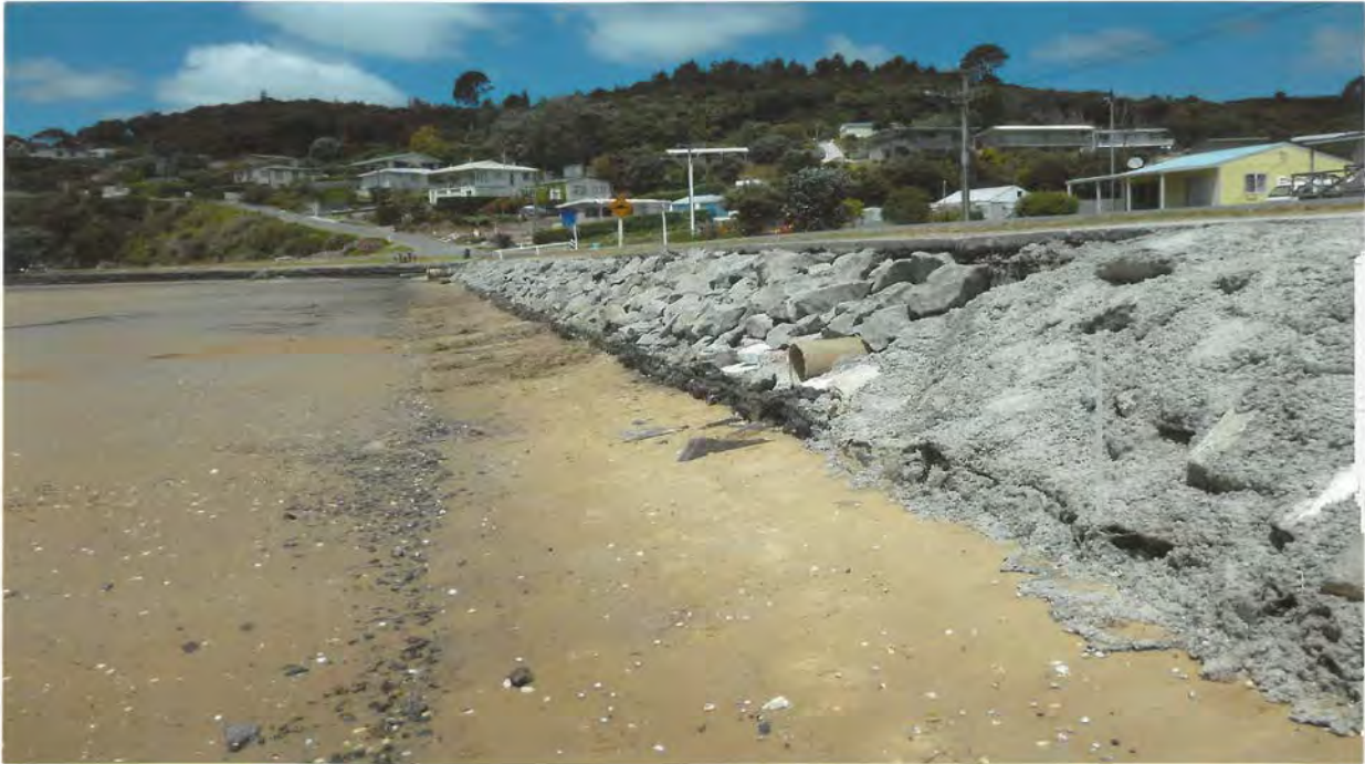
Gabions at Kellys Bay
