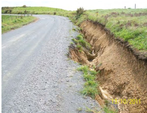
Lawrence Road Improvements before
