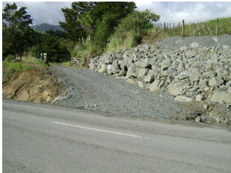
Cleared driveway with rock armour bank
