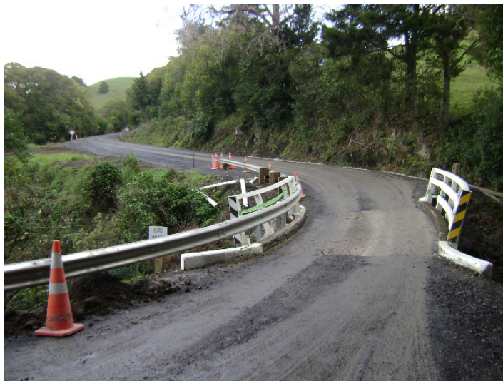
Approach to Omana Road Bridge
