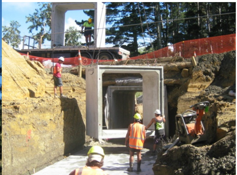
Pukehuia Road Culvert Installation
