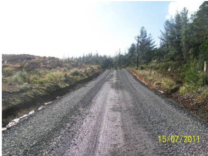
Chadwick Road layer works
