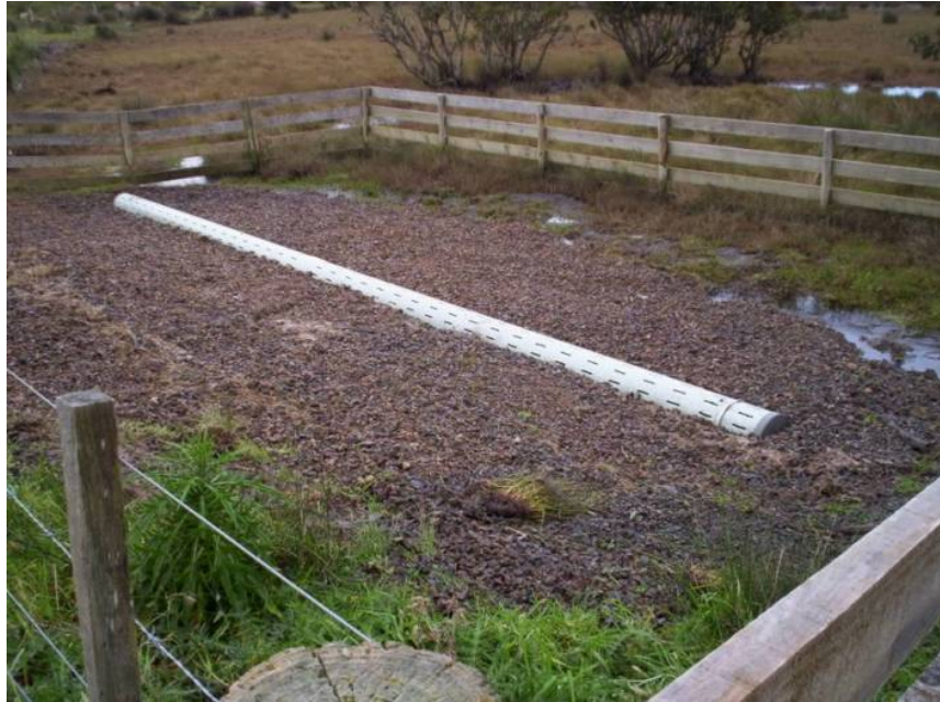
Kaiwaka Wastewater Diffusion Pipeline
