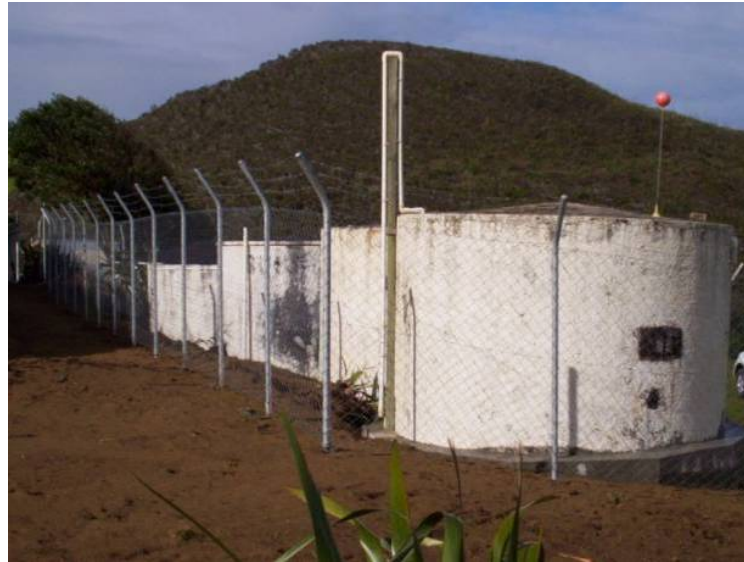
Glinks Gully Treatment Plant newly completed security fence
