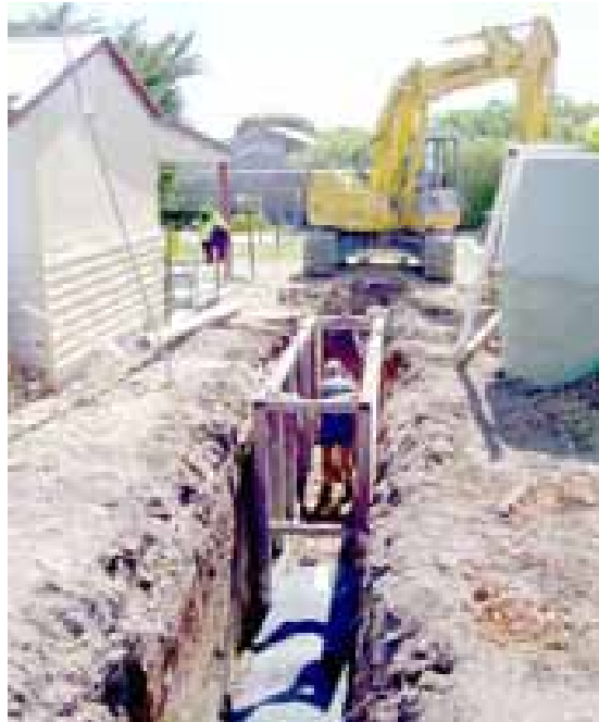
Figure 3-8: Installation of Conventional Gravity Sewer through private land.
