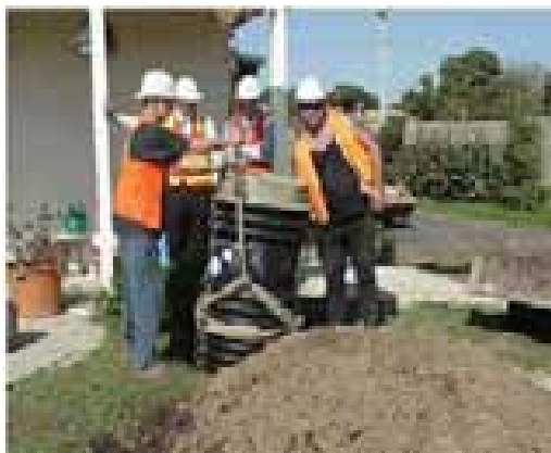
Figure 3-2: Installation of Grinder Pump and Pit
