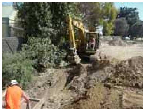
Figure 3-7: Installation of Conventional Gravity Sewer
