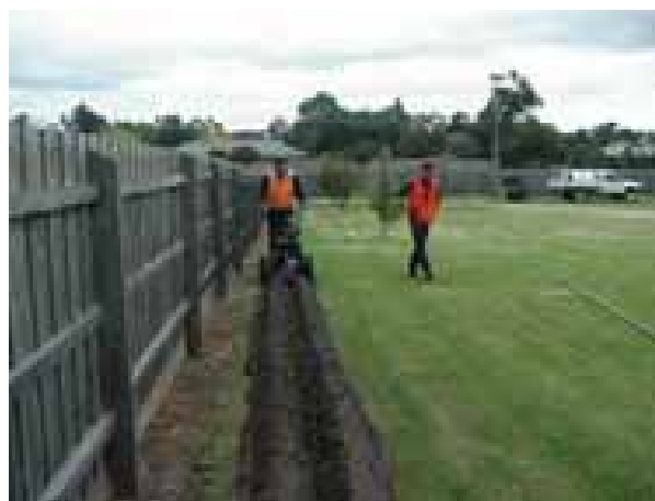
Figure 3-4: Installation of a Low Pressure Sewer Main
