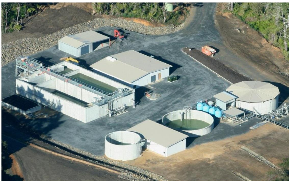
Mangawhai Wastewater Treatment Plant
