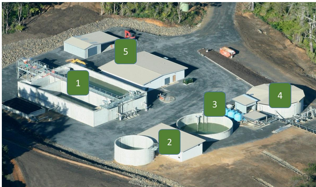
Figure 6-1: Aerial View of MCWWS Treatment Plant
